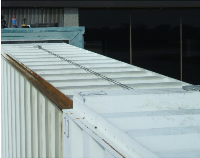
This device is a two cable lifeline with 4 bolt anchors on either end of each tunnel.
